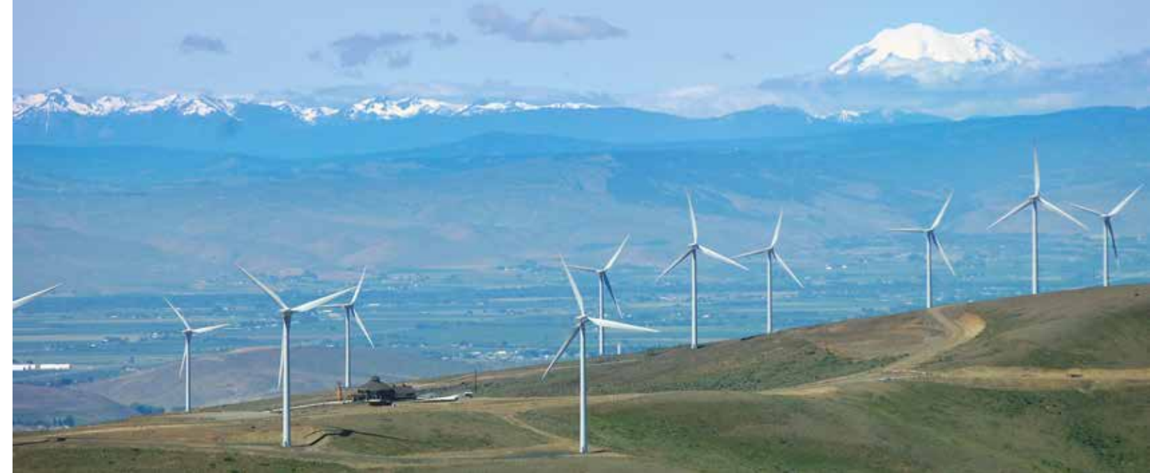
Wild Horse Wind and Solar Facility, photo courtesy Puget Sound Energy.
