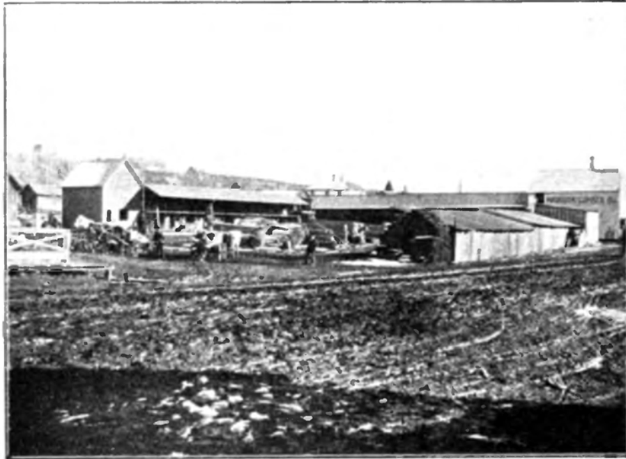
Lumber, Wood and Coal Yard of Madison Lumber Co.
